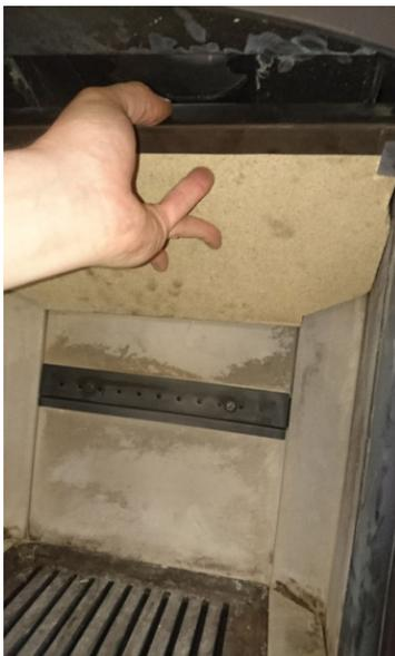
*Lift the throat plate from the retaining brackets and carefully remove.*
