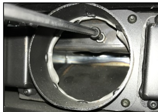
SE Fixing Being Adjusted
