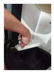
Remove grate and base fire bricks.
