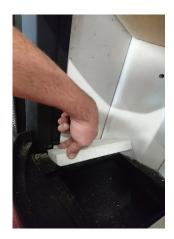
Remove grate and base fire bricks.
