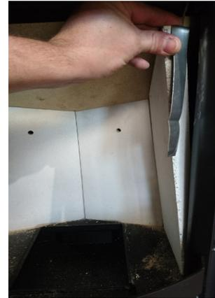
*Carefully lift out both side fire bricks, ensuring the securing clip remains with the brick.*
